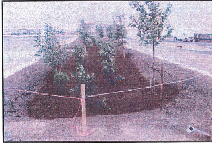
Newly Constructed Bioretention Area
